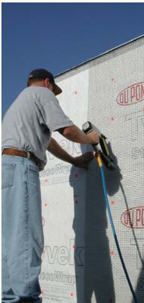
PermaLath can be installed vertically, horizontally and even diagonally.
