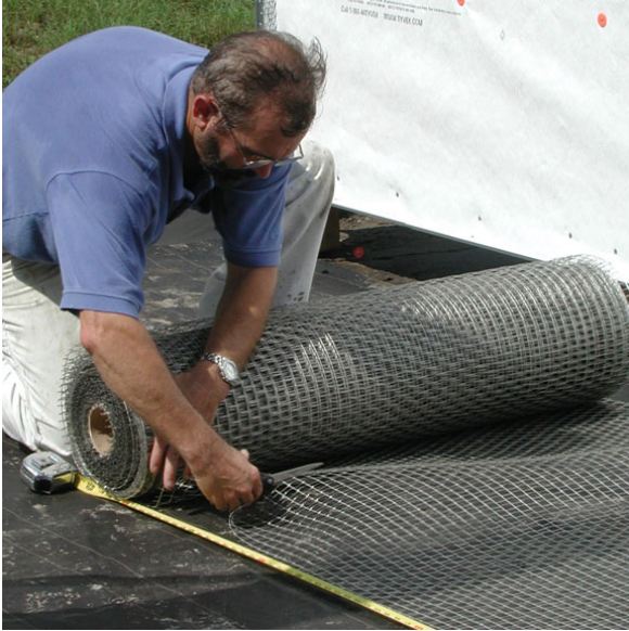
(Caption) PermaLath 1000 application – cutting pieces with scissors or utility knife.
