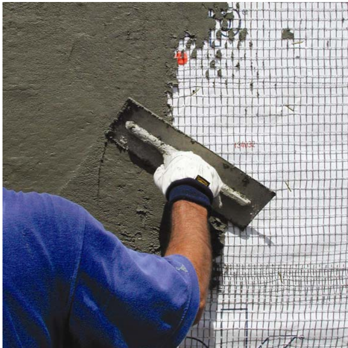
(Caption) Self – furring fiberglass composition will not corrode
